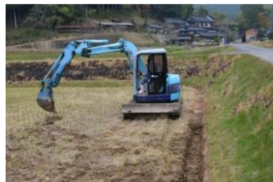
Open channel construction work using a backhoe
